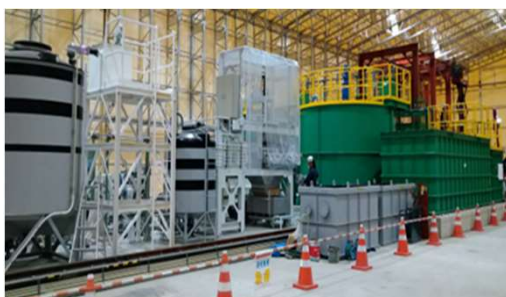
Cleaning process equipment
